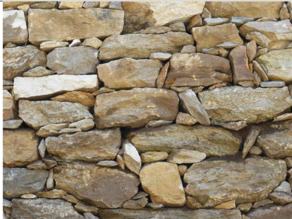
Typical dry stone masonry that imparts flexibility to withstand seismic shocks
